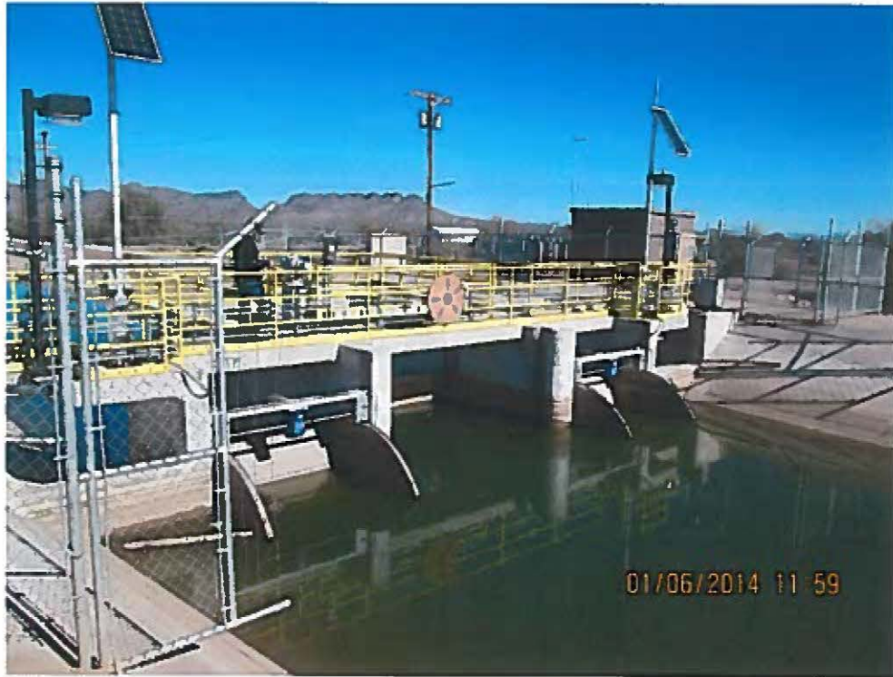
Figure 5 – Typical Radial & FlumeGate Configuration at P-MIP
