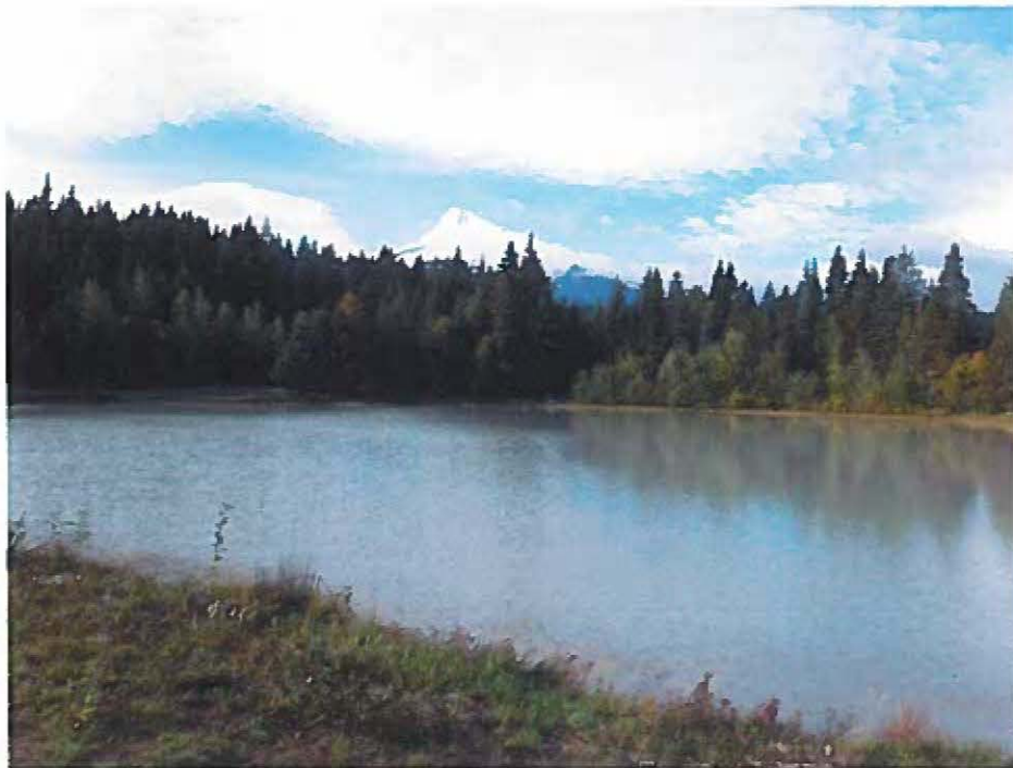
Figure 1: MFID's existing settling basin enables removal of glacial sediment from irrigation water
