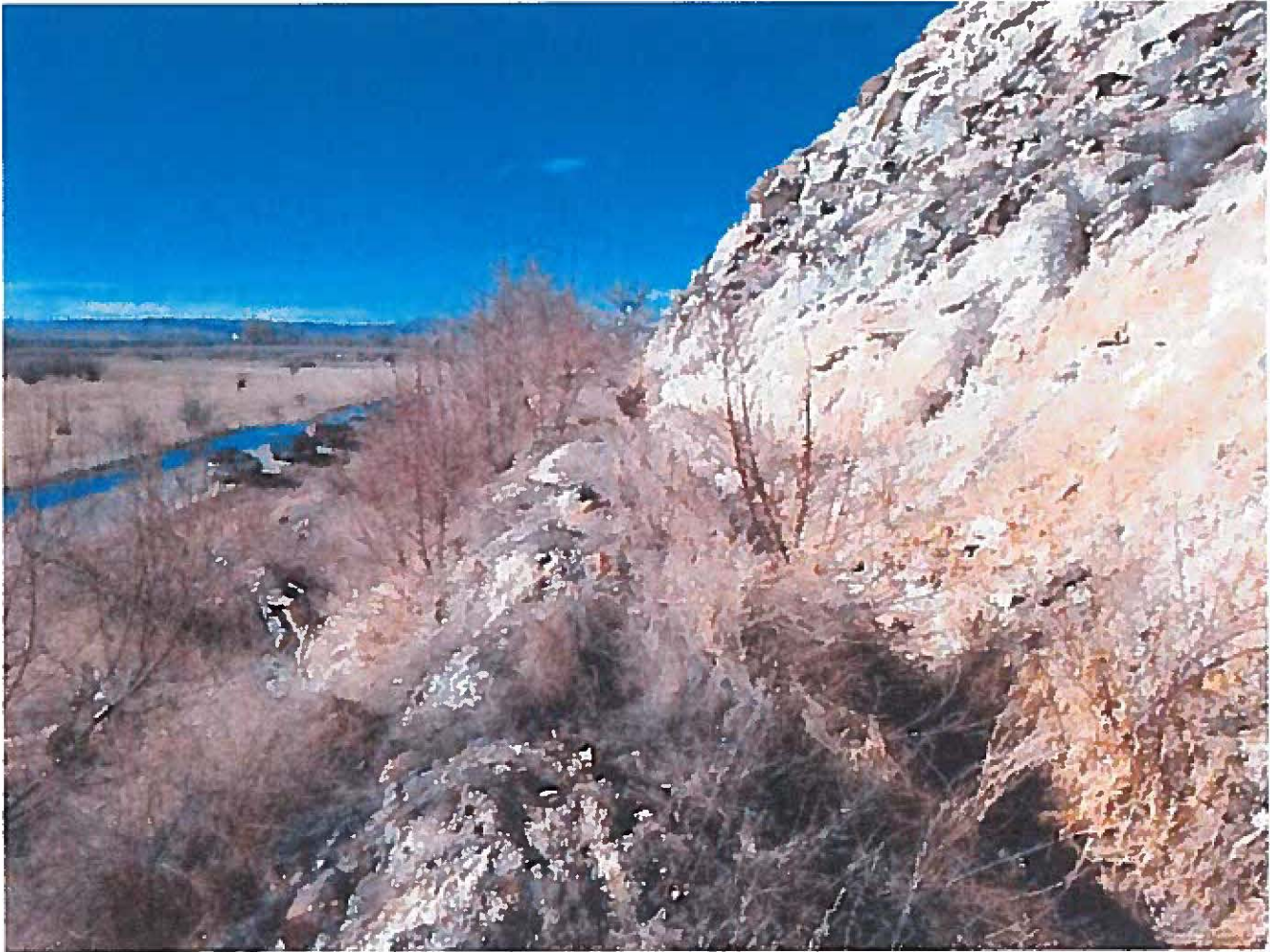
Figure 1: Lower Reach Slide Area
