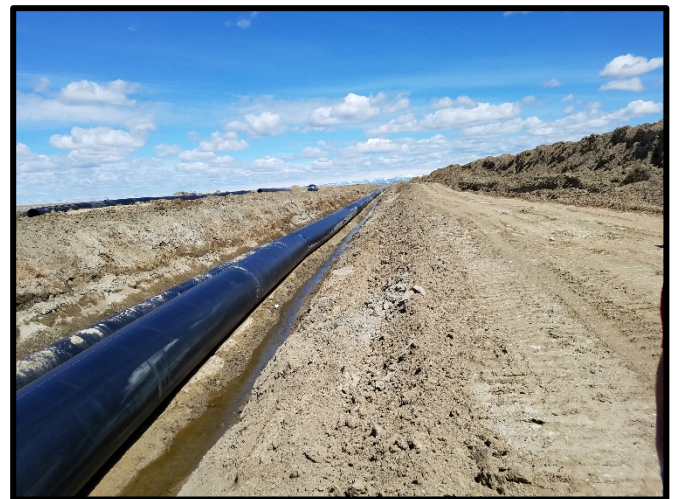
Photo 3 Farson Phase I Completed in 2016
