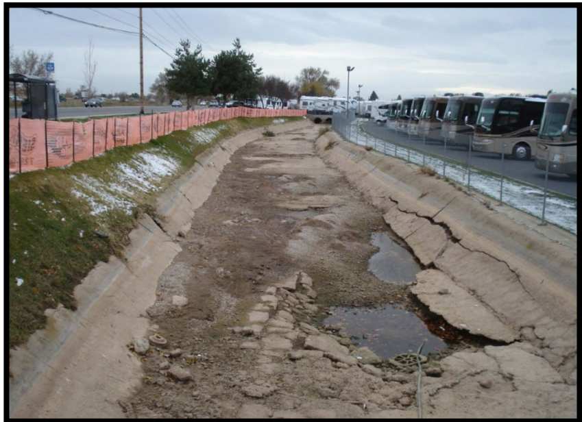
Photo 1 Unlined Canal in Front of U-Haul Business
