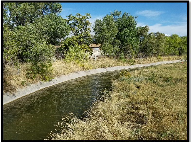
Photo 2 Open Canal Near Homes
