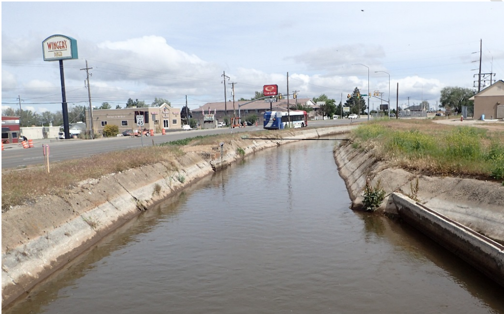
Figure 9 - Downstream measurement location. Black line indicates approximate location of measurement.
