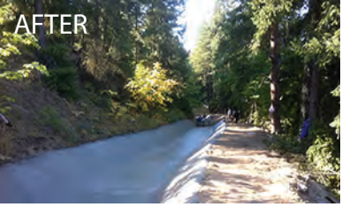
BEFORE AFTER LINER REPLACEMENT
