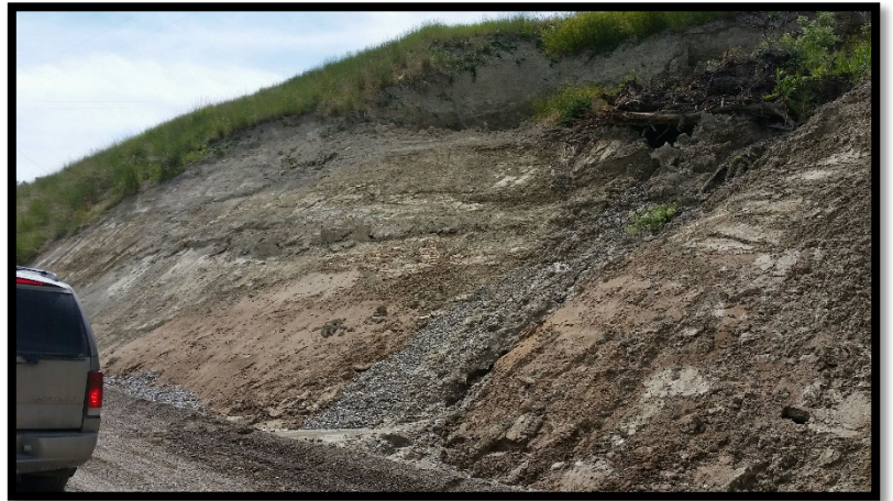
Photo 2 Hillside with soil and rocks slipping away
