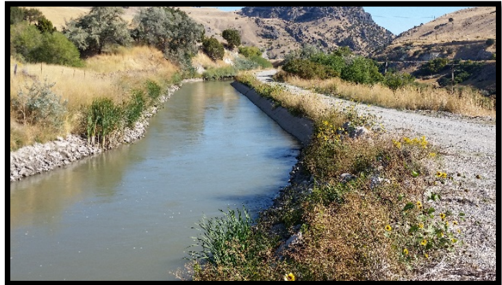
Photo 2 West Main Canal
