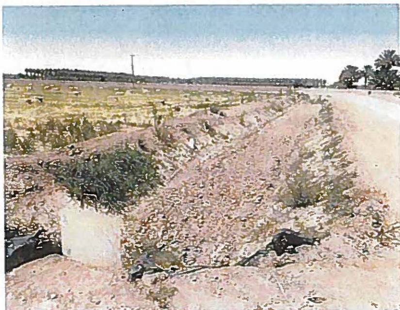
Image 1. Bard, CA. Example of earthen irrigation ditch.
