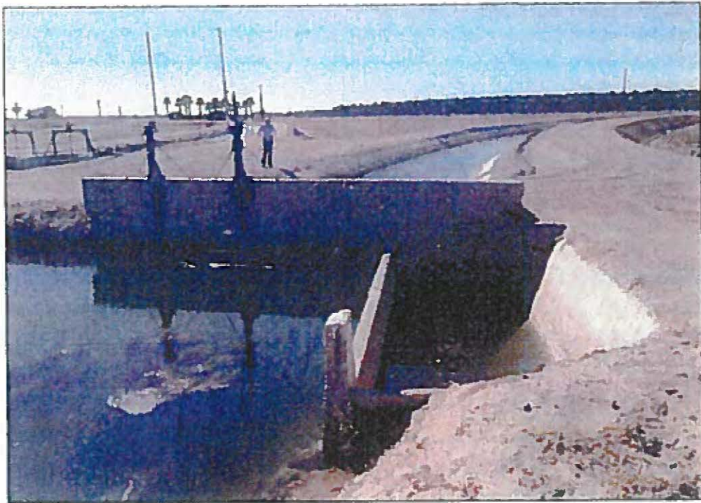
Figure 12.—Gate #5 in Five Gates is an overflow culvert.
