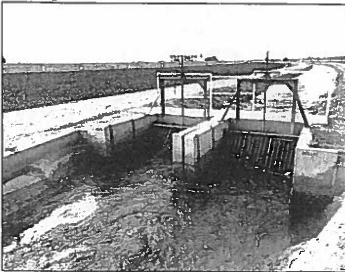
Mojave canal diversion at Reservation Main Canal. BOR photo
