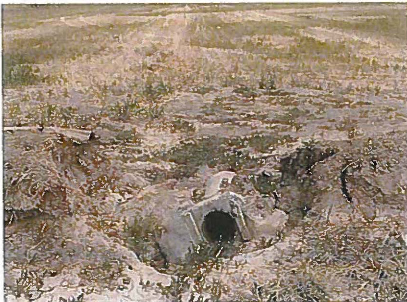
Image 3. Bard, CA. Example of distribution port in collapsed earthen embankment.
