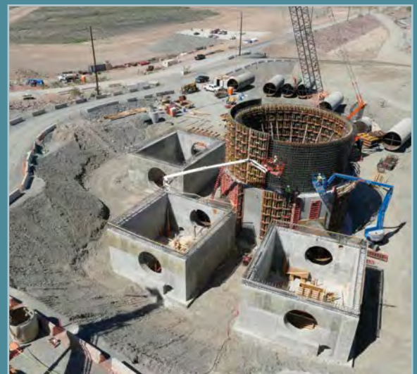
Low Level Pumping Station Construction
