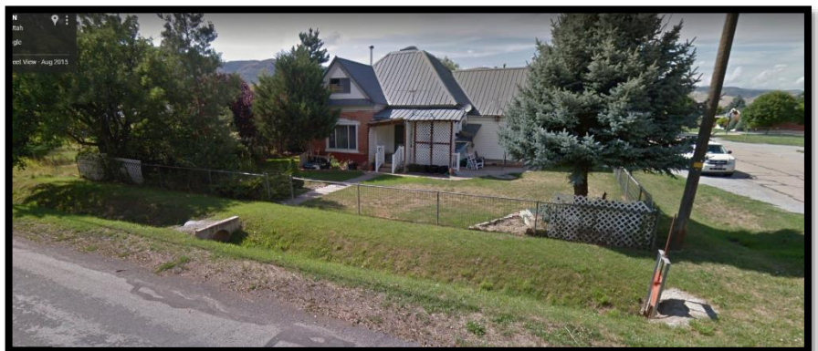
Photo 5 Open Middle Town Ditch
