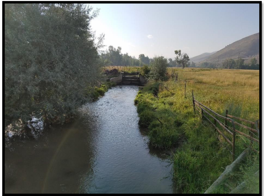
Photo 4 Main Ditch Unlined
