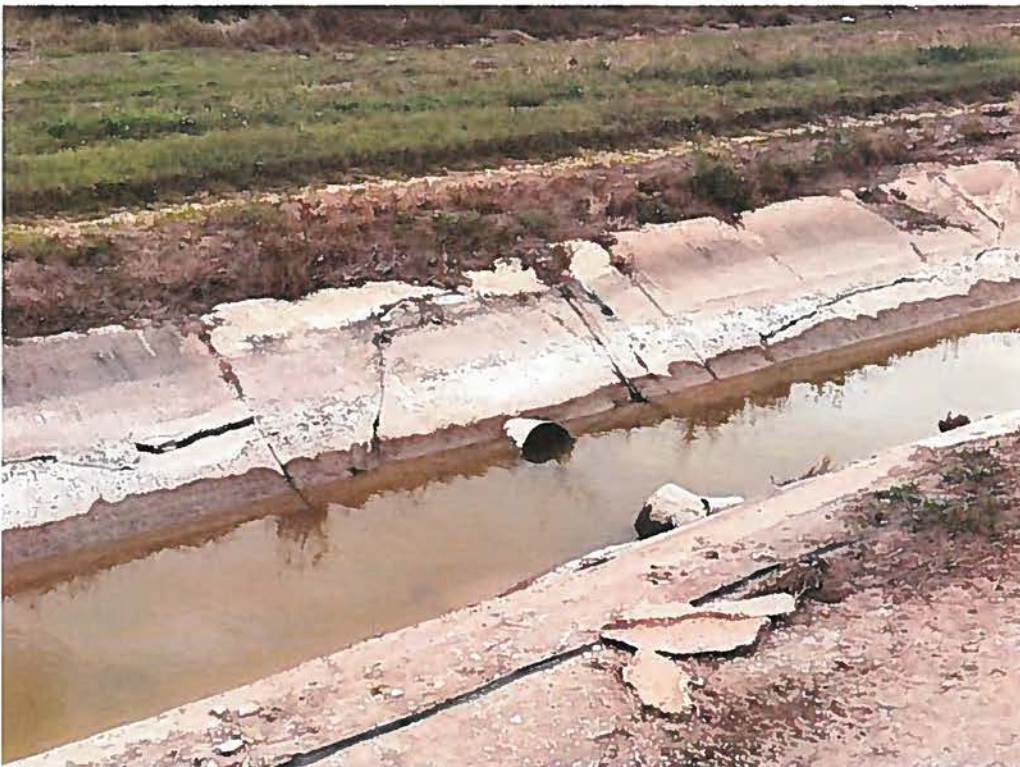
Picture 5. Typical field outlet pipe laterals.
