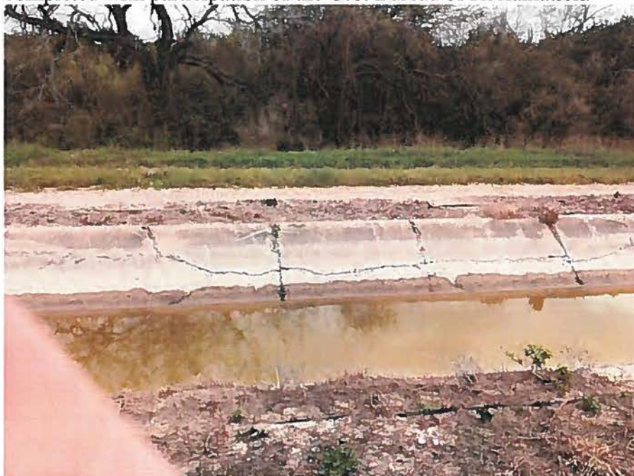
Picture 1. (Background) Visible horizontal crack in the east side slope. Horizontal cracks extend for the entire canal length on both interior side slopes.
