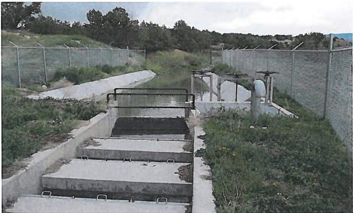
Figure 5. Sluice Structure, End of Canal
