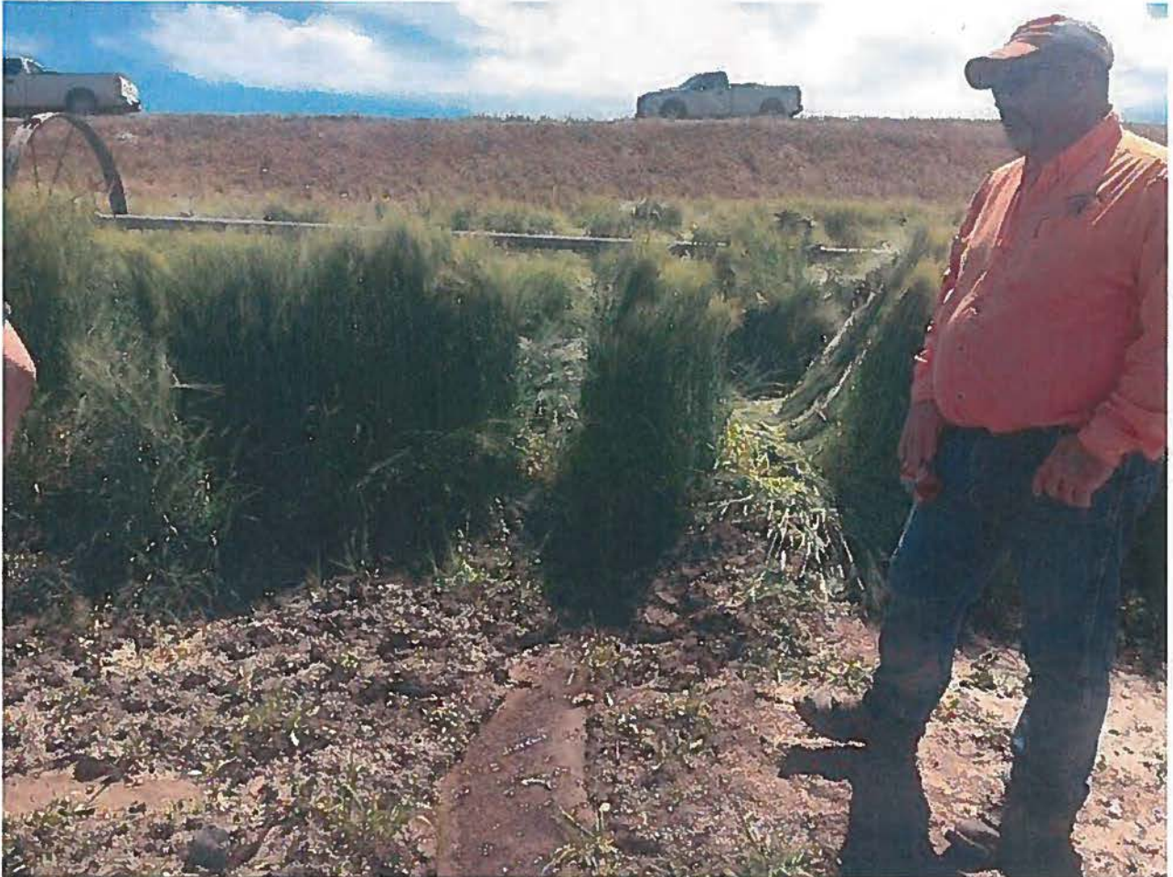
Figure 5. 2018 Canal Seepage Resultant from Damage to an Existing Drain Tile
