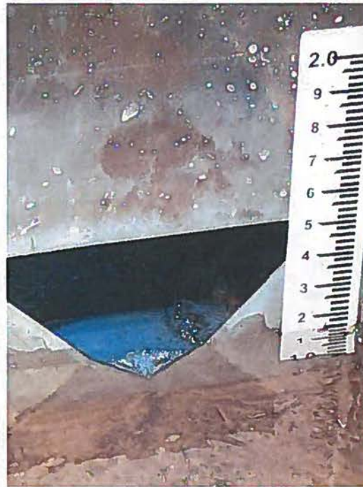
Figure 6. Flow Measurement Weir Installed to Quantify 2018 Canal Seepage Resultant from Damage to an Existing Drain Tile
