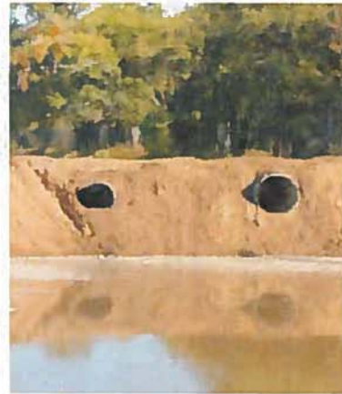
Canal seepage loss ponding test, Franklin Canal, El Paso, Texas
