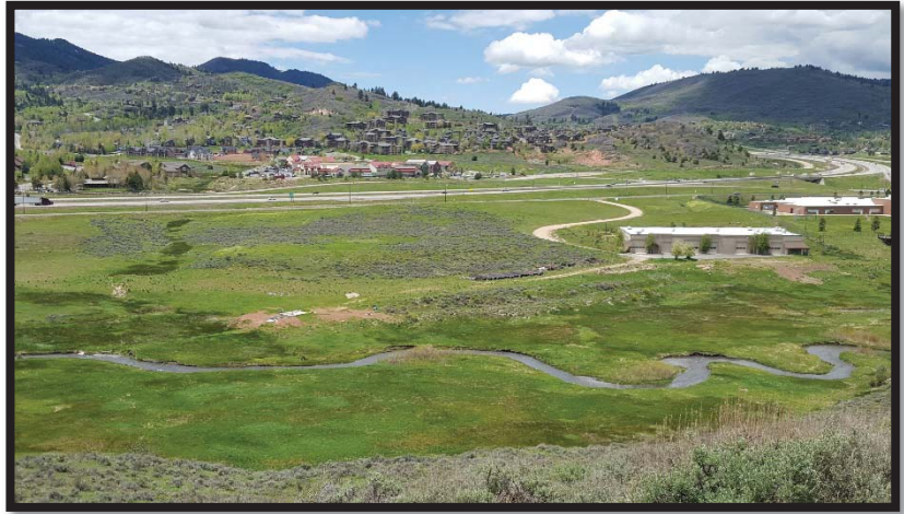
Photo 1 East Canyon Water Treatment Plant
