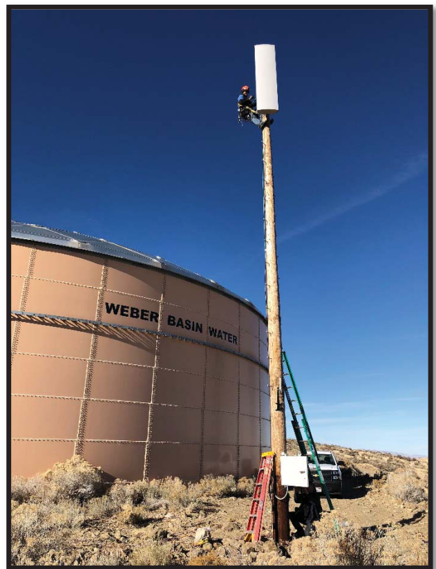
Photo 2 Little Mountain Water Tank
