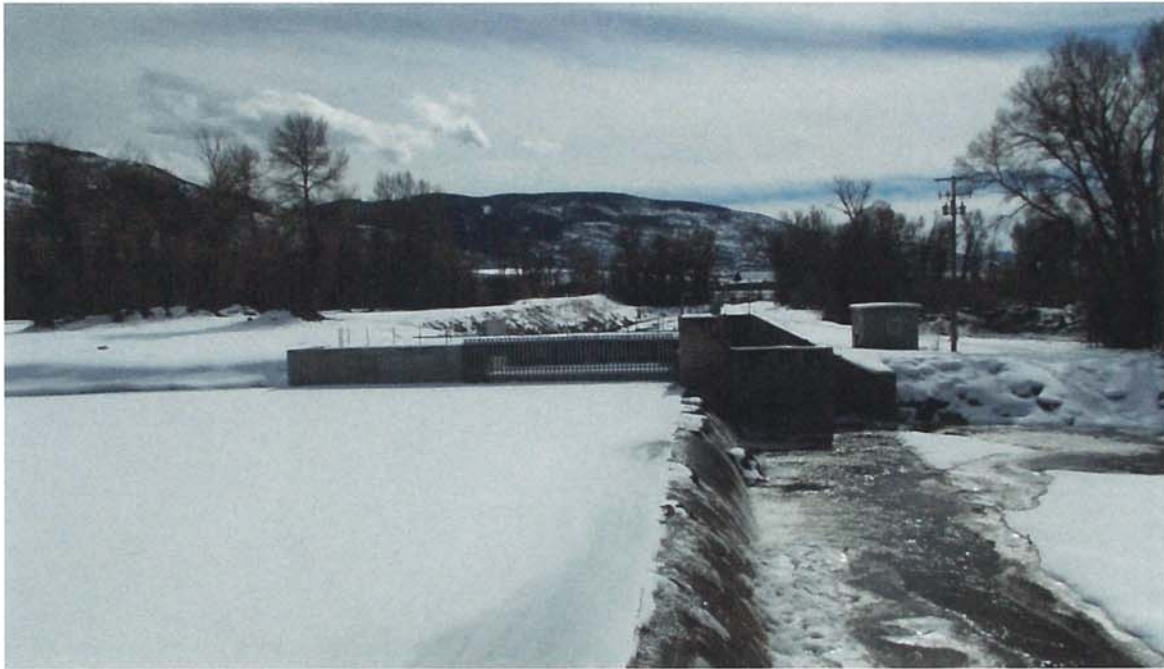
Figure 3 – Weber-Provo Diversion Dam (winter conditions)
