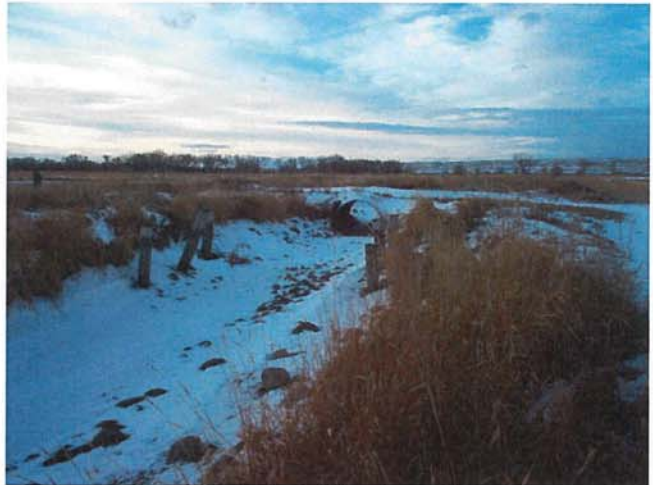
12/18/2013 IM000461.JPG Looking West (Upstream) from Near Siphon Inlet
