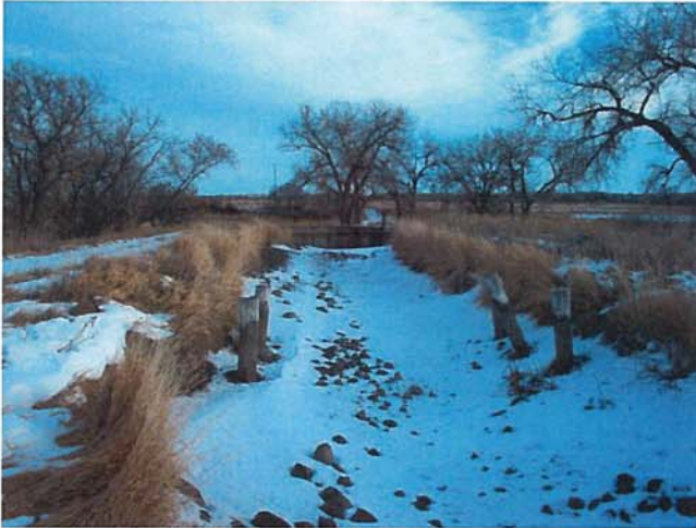
12/18/2013 IM000460.JPG Looking East (Downstream) Towards Siphon Inlet
