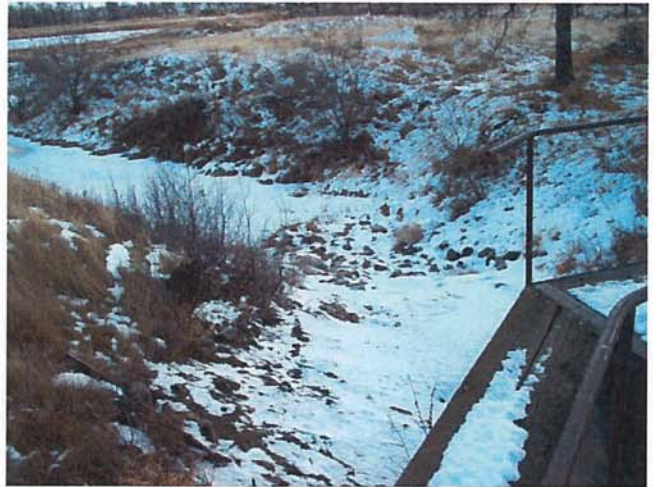
12/18/2013 IM000465.JPG Looking East (Downstream) at Wasteway Channel
