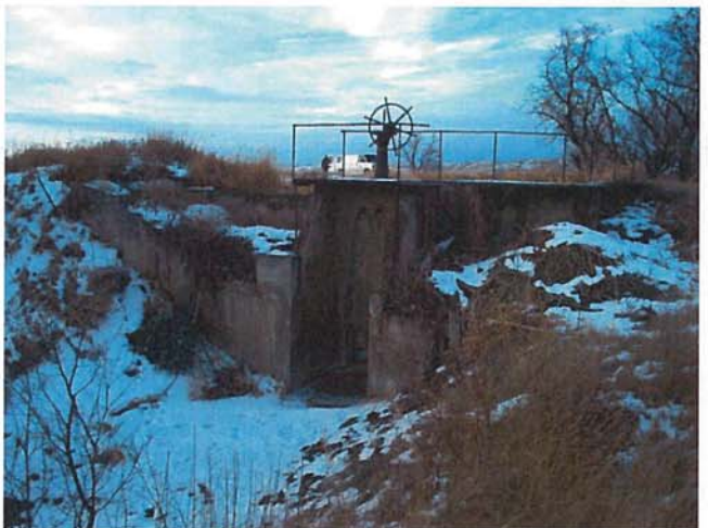
12/18/2013 IM000467.JPG Looking West towards back of Wasteway Gate and Overflow Weir
