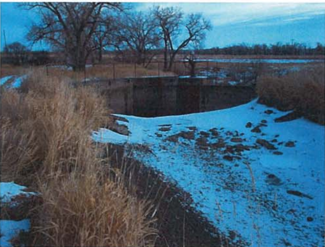
12/18/2013 IM000462.JPG Looking East (Downstream) Towards Siphon Inlet
