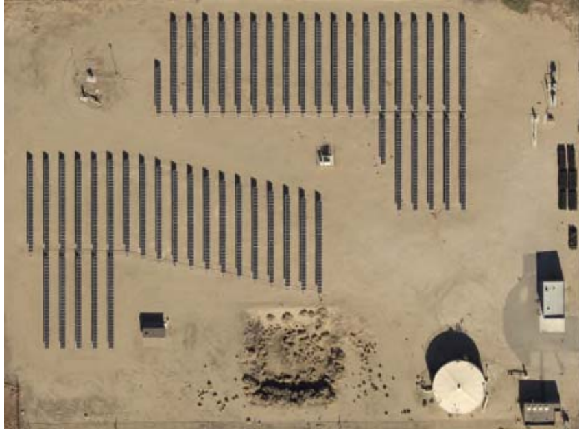
Figure 1-2: Avenue K and 5th Street West Solar Field
