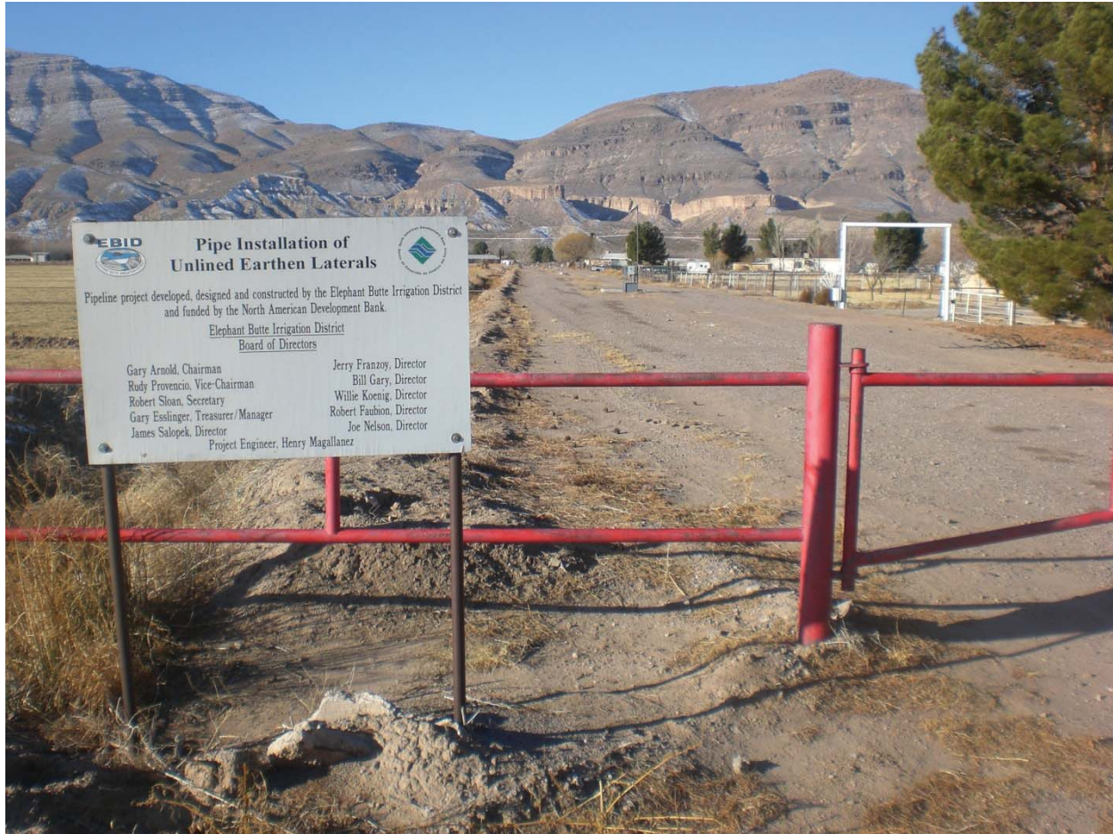
Figure 4: The Kerr Lateral, which has been placed in pipe.
