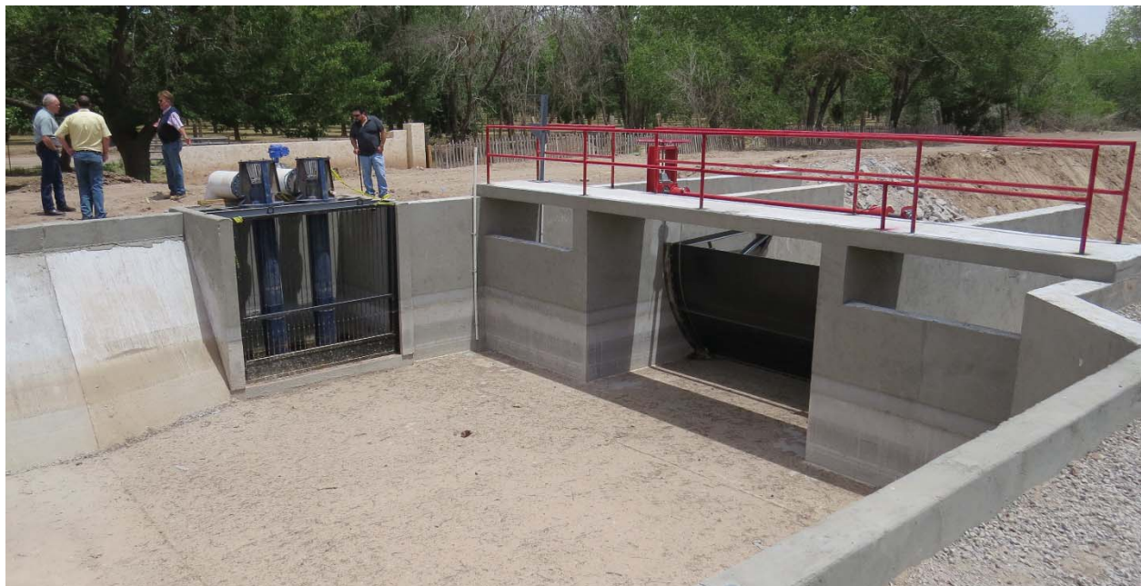
Figure 2: Lift pump on the Eastside Canal conveying water from the head of the Mesilla Dam diversion to the tail end of the Leasburg system.
