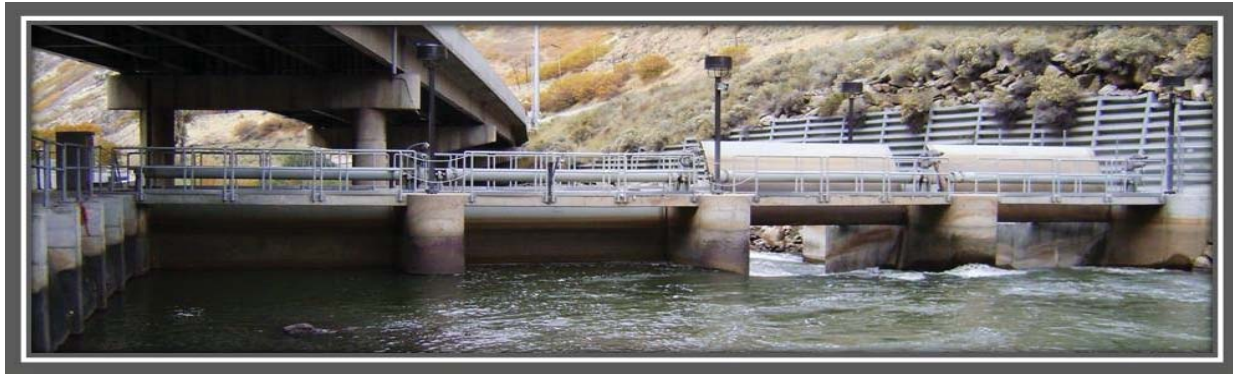
New Headwork's Structure Funded with Challenge Grant Funds
