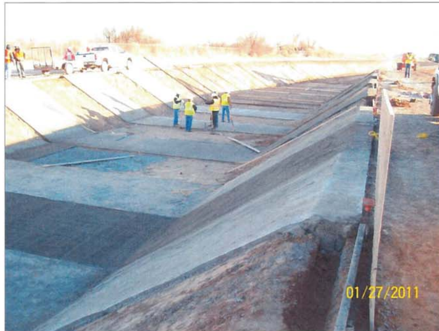
FIGURE 4 Typical Construction of Shotcrete-Lined Canal
