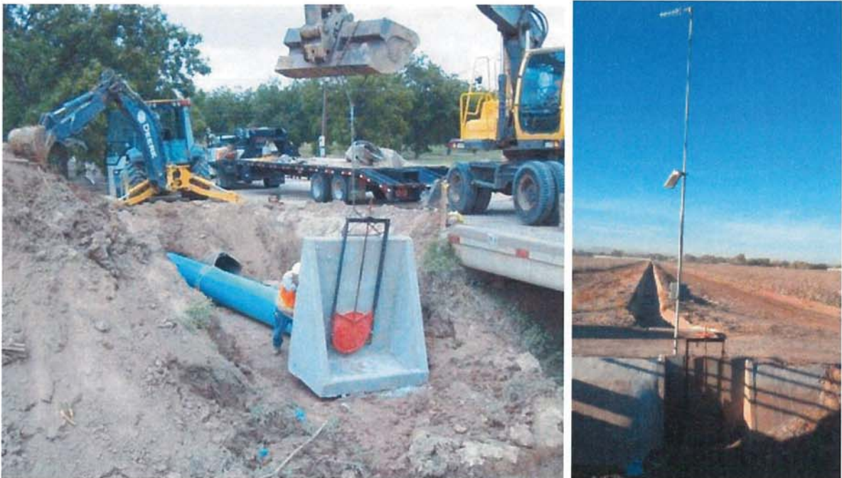
FIGURE 14 2012 Project: Installation of Headwalls and Telemetry Units
