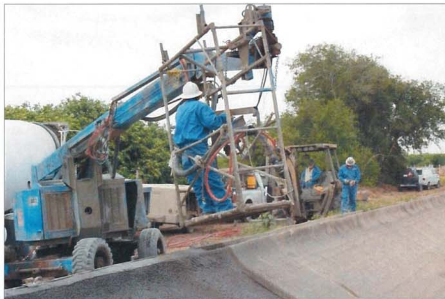
FIGURE 5 Typical Equipment for Shotcrete Application
