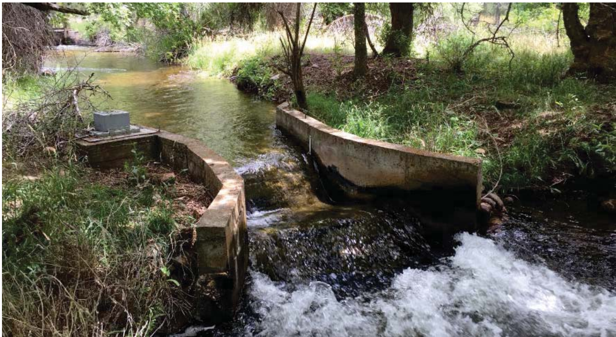
Figure 2. Photo of Site 1 measurement location.
