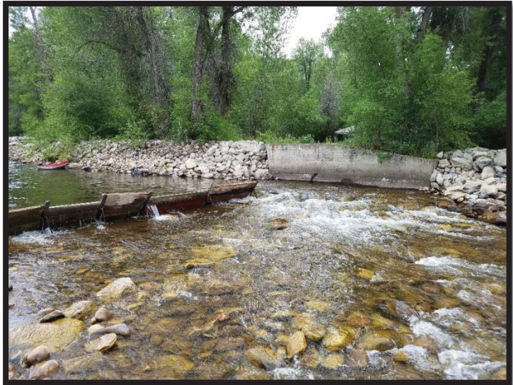
Photo 1 Weber River Diversion for South Bench
