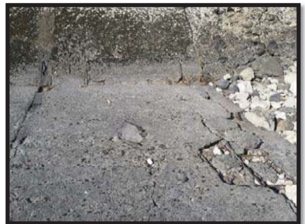
Photo 4 Exposed Rebar
