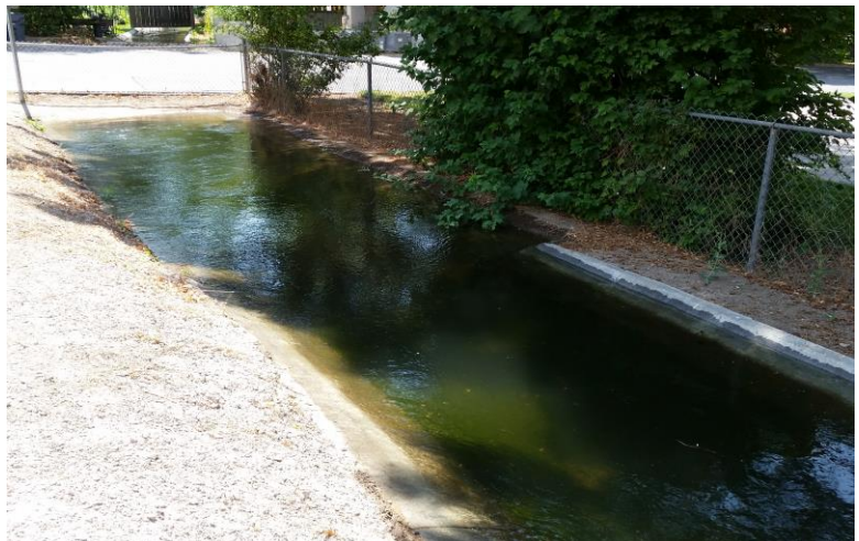
The canal does not have the capacity to carry the full water right and water is lost as it spills over the bank.
