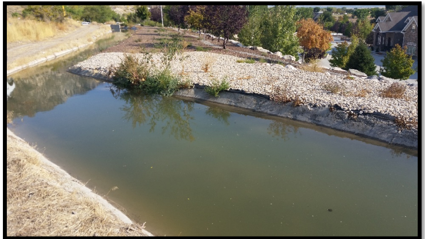
Photo 3 Hammond East Canal Above Homes
