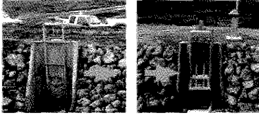
Remove existing manual gate and... replace with face mounted SlipMeter™
