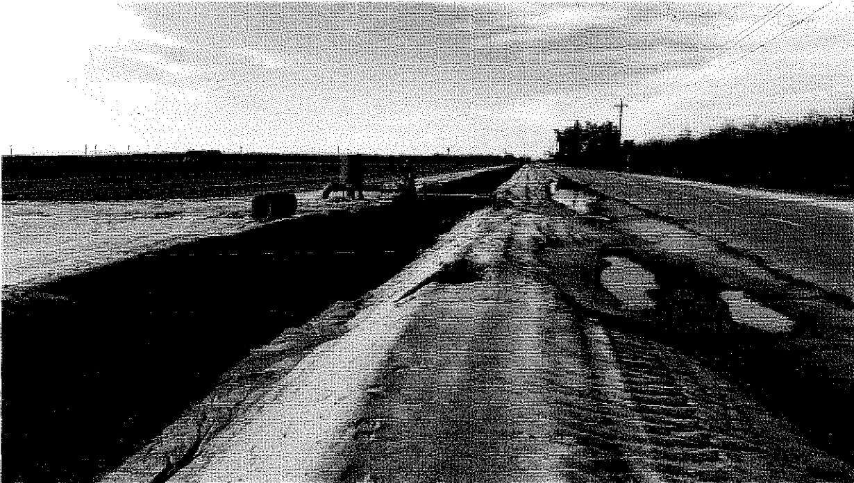
Existing breach through canal bank. Roadside puddles and none in sandy canal.
