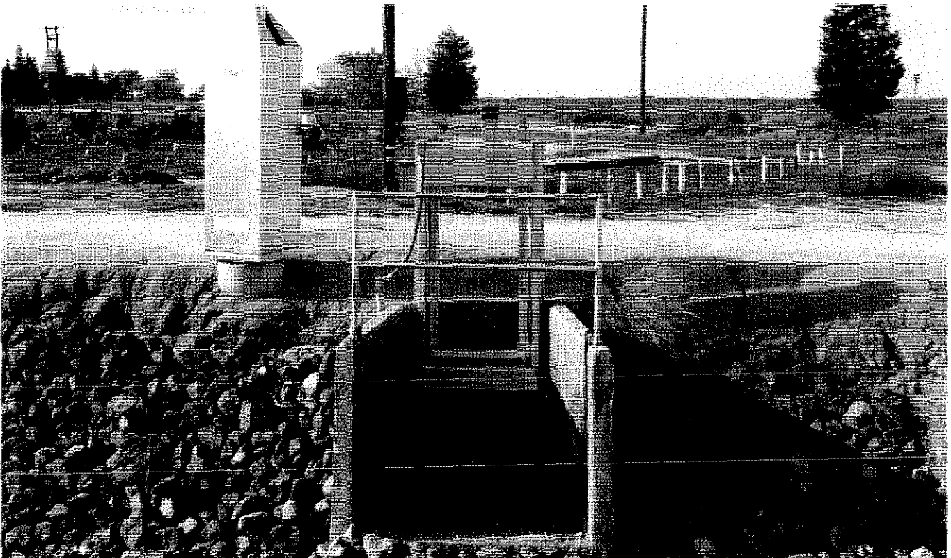
Example of new Automated Slip Meter connected to SCADA system
