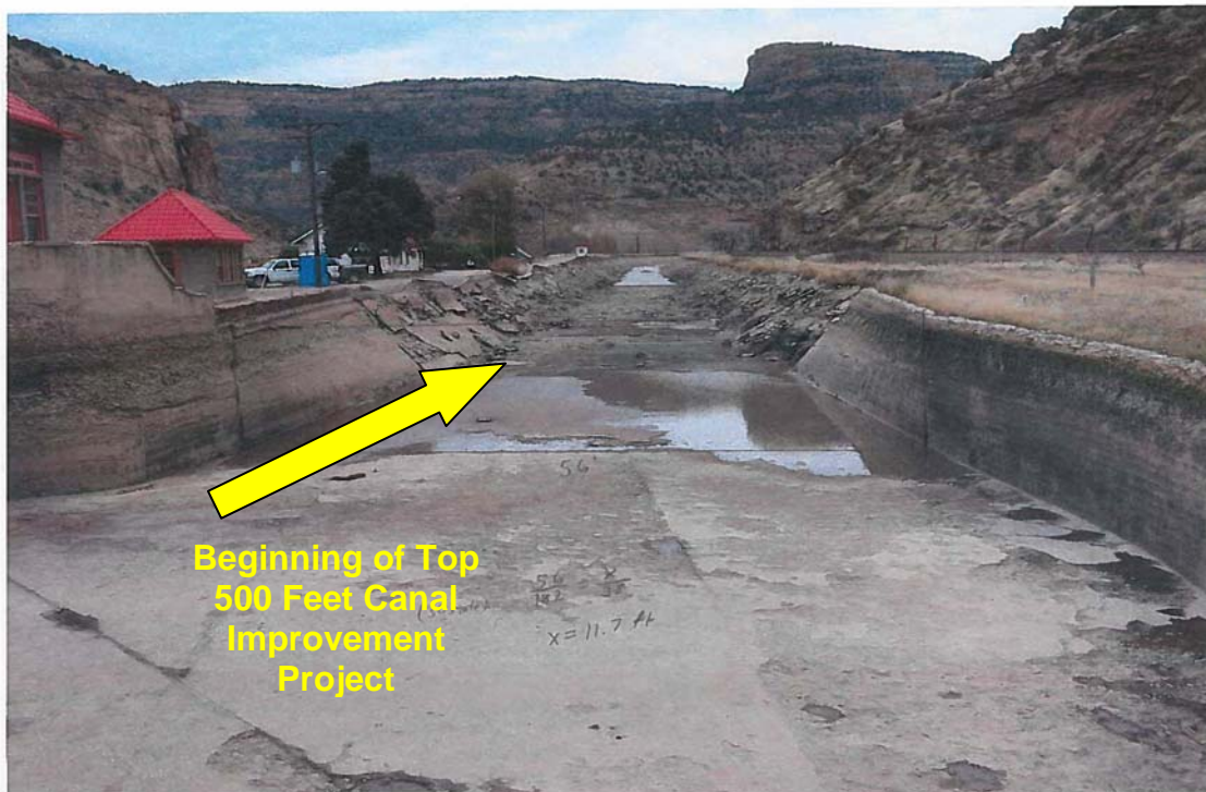
Figure 5. General setting and existing condition of the top 500 feet of the Canyon Canal; looking down canal.
