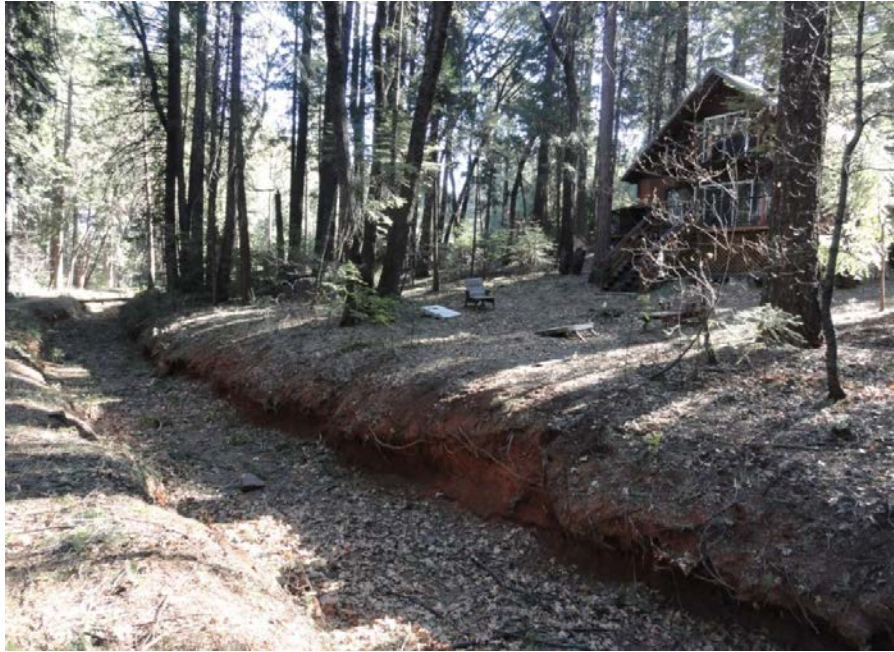
Photo 2 – Erosion along Ditch Alignment with Rock Stabilization
