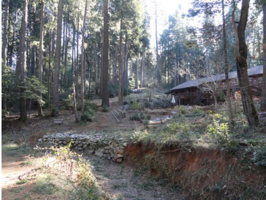
Photo 2 – Erosion along Ditch Alignment with Rock Stabilization
