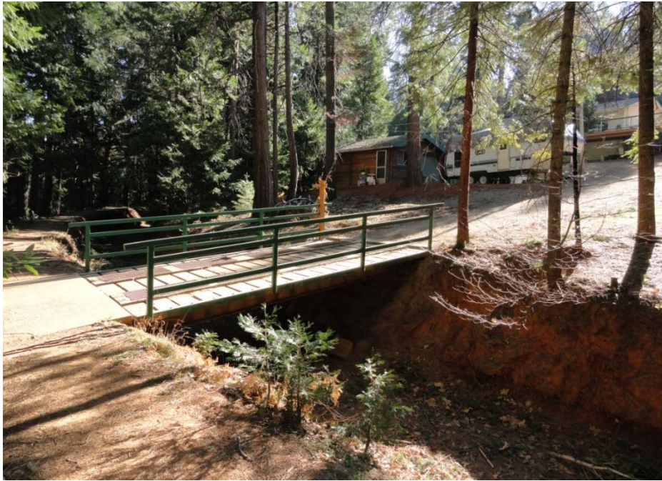
Photo 4 – Bridge Crossing – Erosion Jeopardizing Abutments
