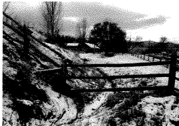
Unlined ditches create water loss through seepage and continual maintenance issues.
