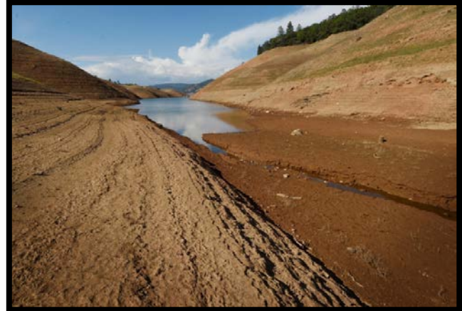
Fig. 4: The California drought has exposed the bottom of Oroville Lake reservoir which is now at 26% of its capacity.
