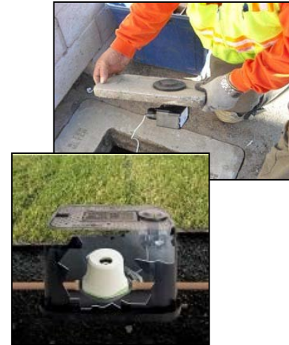
Fig. 1: Example of an AMI transponder attached to a water meter.
