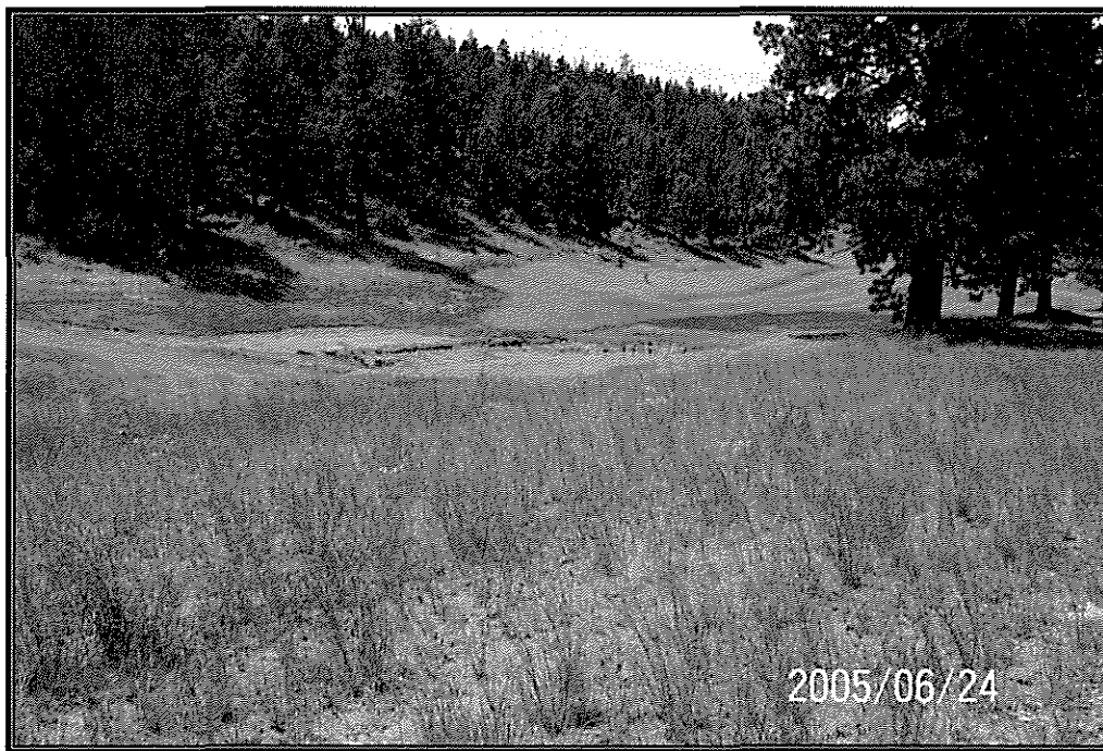
Figure 3: Typical Post-Construction View of Buried Pipe Alignment, From Bend Feed Canal Piping Project.
