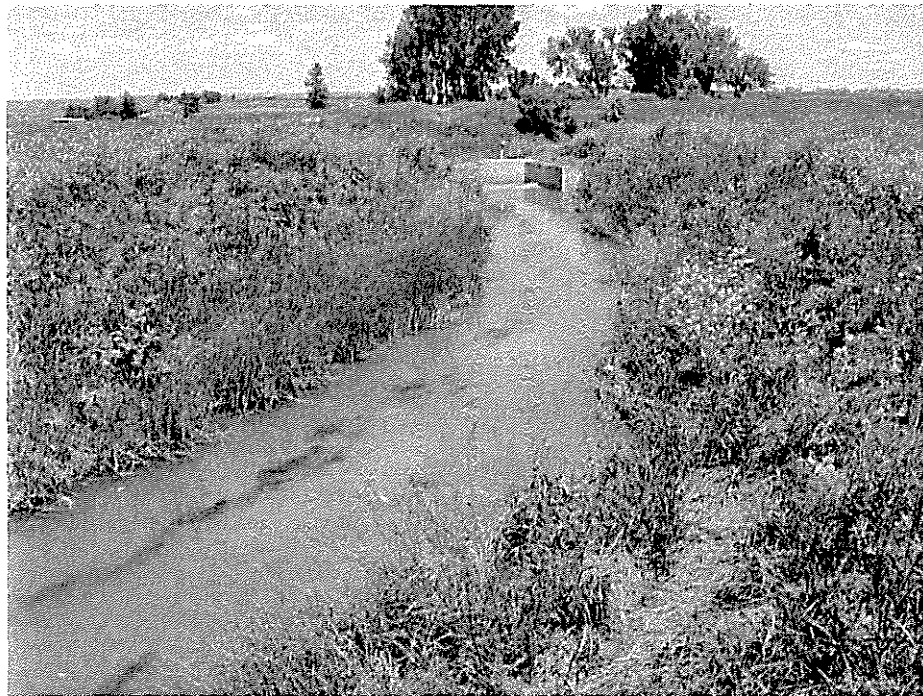
Photo 2 - High Canal at 1500 feet showing the beginning of moss and algae vegetation growing in the middle of the canal.
