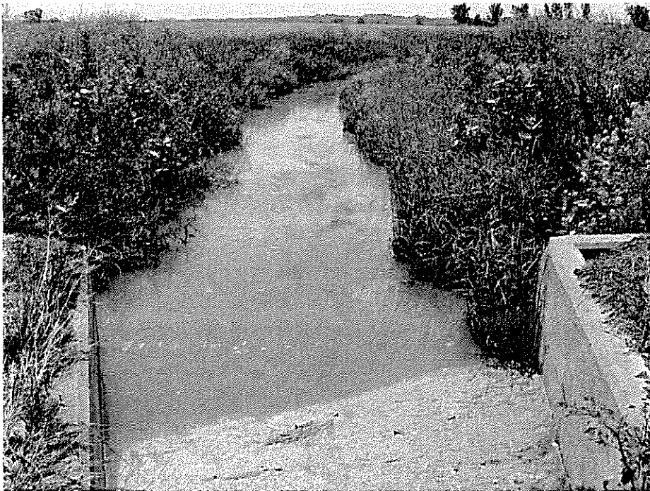
Photo 4 - High Canal at the siphon showing moss and algae growing in the water and floating debris caught up. Infestation of noxious weeds covering the banks.
