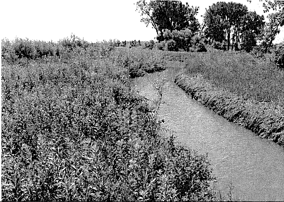
Photo 5 - High Canal winding around the high side of the contour elevation bench change.
