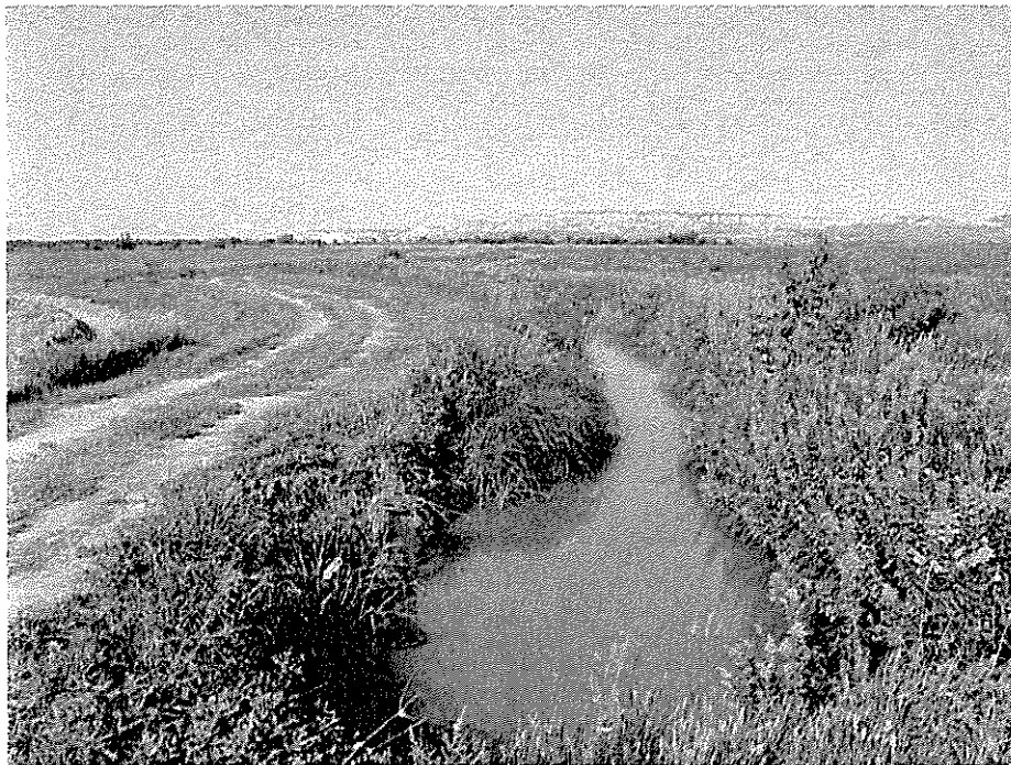
Photo 14 - High Canal heading east to the end. Showing weeds and vegetation growth with very slow water flow.
