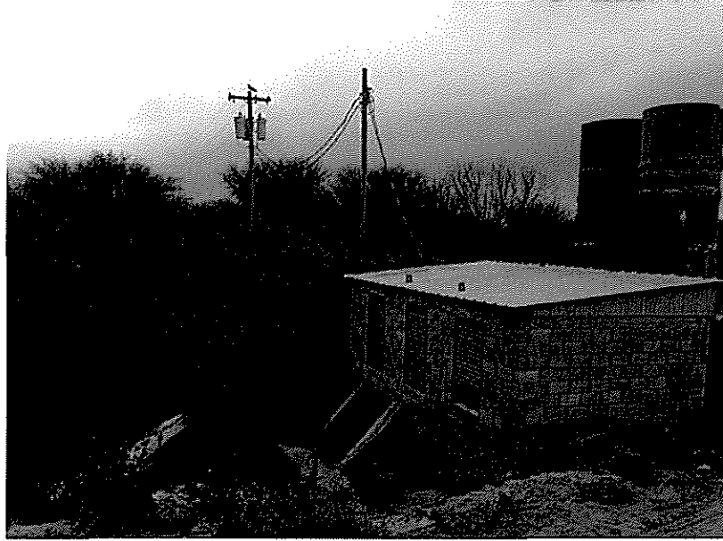
Figure 3.2 Existing Pump-15 Lift Station
