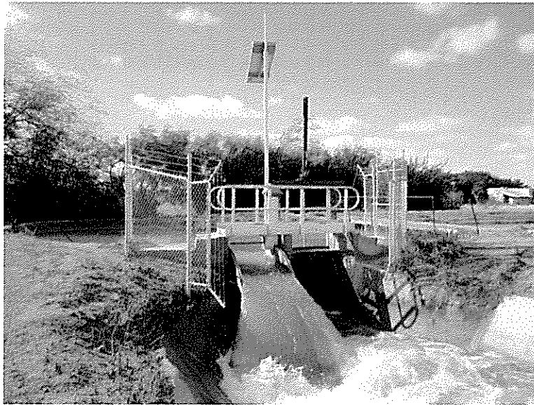
Alamo Main Canal Head Gate (Station 0+00) viewed from the North.
