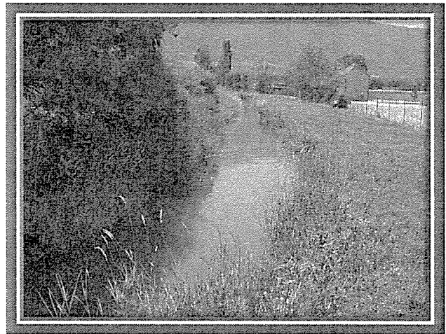
Section of open canal in the delivery system
