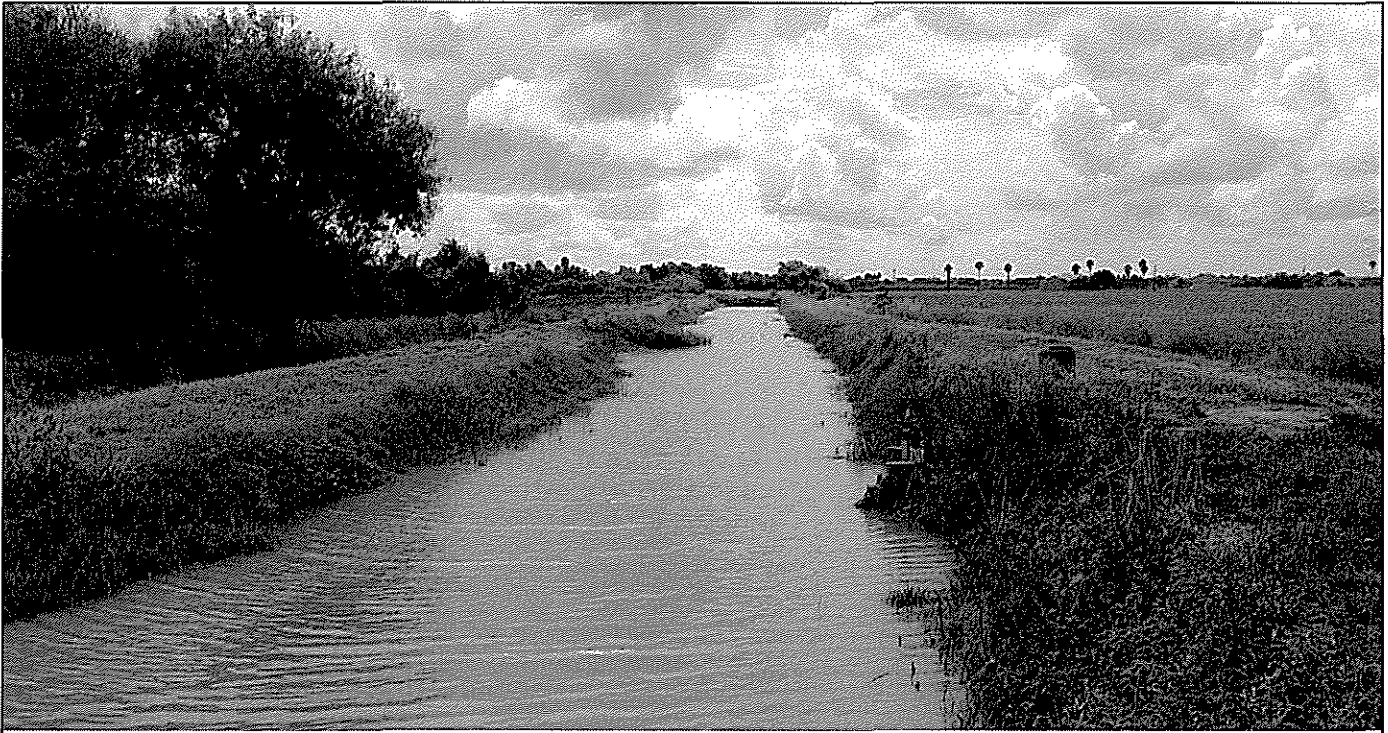
Figure 2.3 Saldafia Canal on Date of Test
