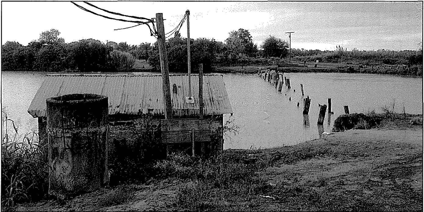
Figure 3.3 - Saldaña Pump Station - Exterior
