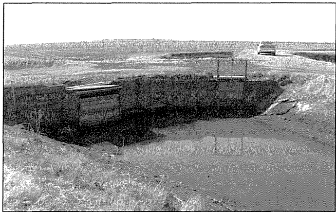
Existing Check Structure and Turnout to R Drain Canal
