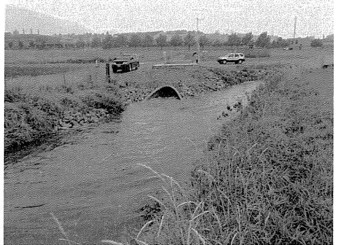
Location where the Piping & Pressurization Project will connect to the Cache Water Restoration Project
