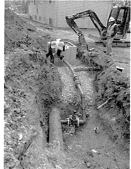
Metered turnout under construction
