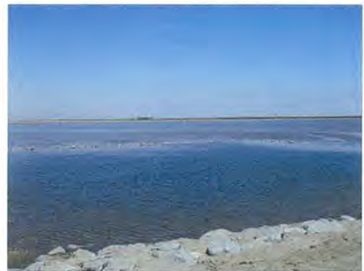
Figure 7: Existing Stockdale West Ranch Recharge Basins
