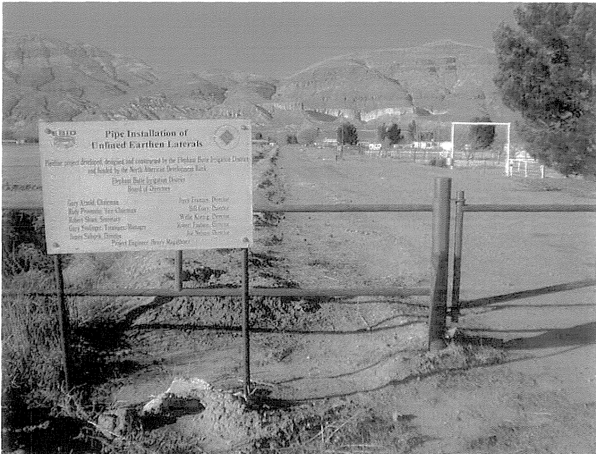
Figure 3: The Kerr Lateral, which has been placed in pipe.
