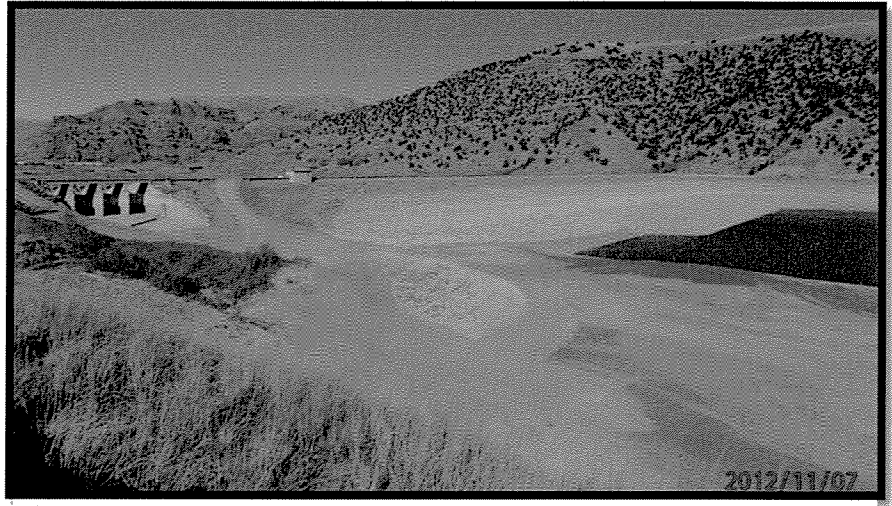
Work on the Echo Dam 2012
