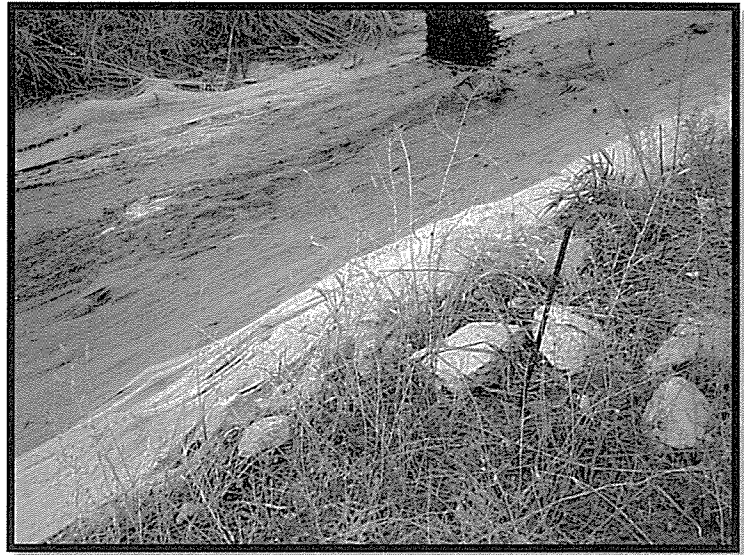
Photo 1 Areas of the canal are currently lined with a type of plastic liner
