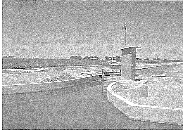
Figure 7. Example of a flow control structure built on the Temple Santa Rita Canal
