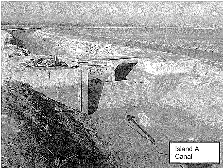
Figure 13. Check #C - Island A Canal.
