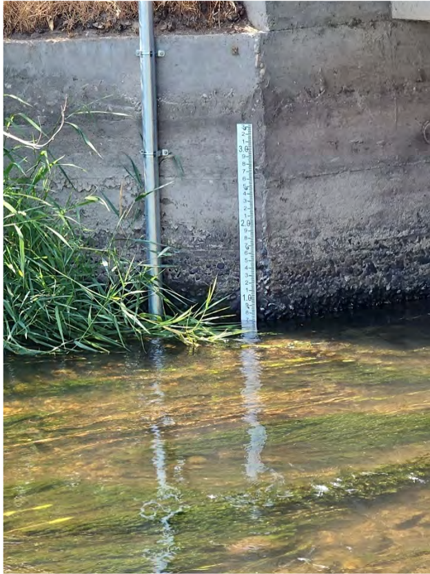
Photo 5 – Examples of water fluctuation at RTM sites installed by the District.
