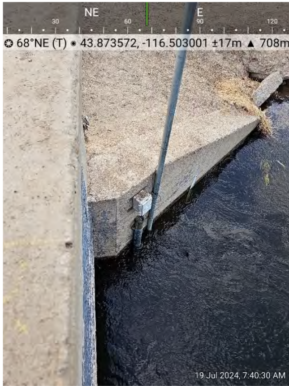
Photo 1 – RTM technology previously installed by District personnel.
