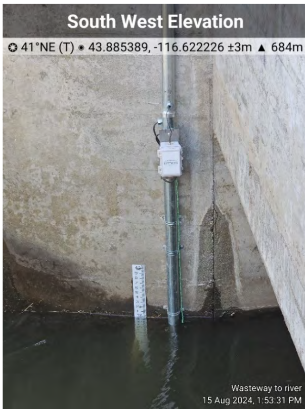
Photo 4 – Several configurations are possible for the RTM technology and the Ethos Connected Telemetry units.
