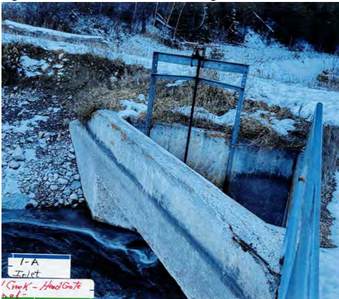
Figure 1-Gate 1-A Town Canal Headgate
