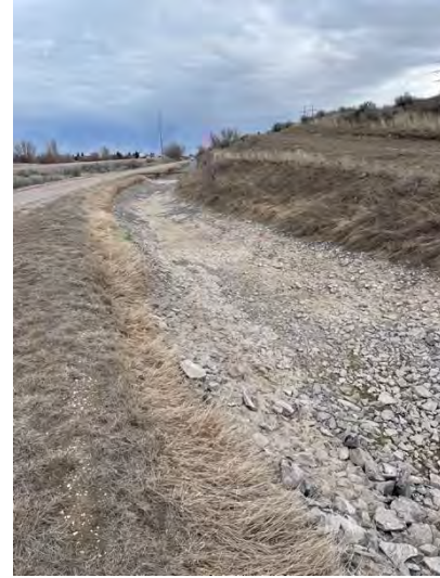
Figure 4 Downstream View from Project Site
