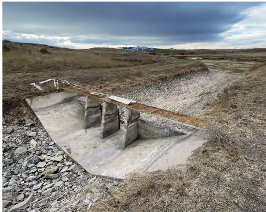
Figure 2 Proposed FlumeGate Automation Project Site
