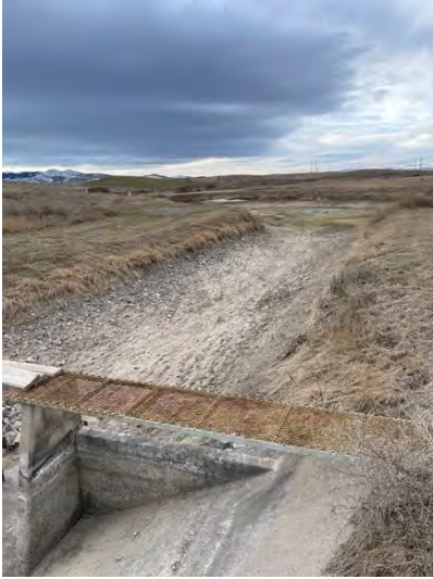
Figure 3 Upstream View from Project Site
