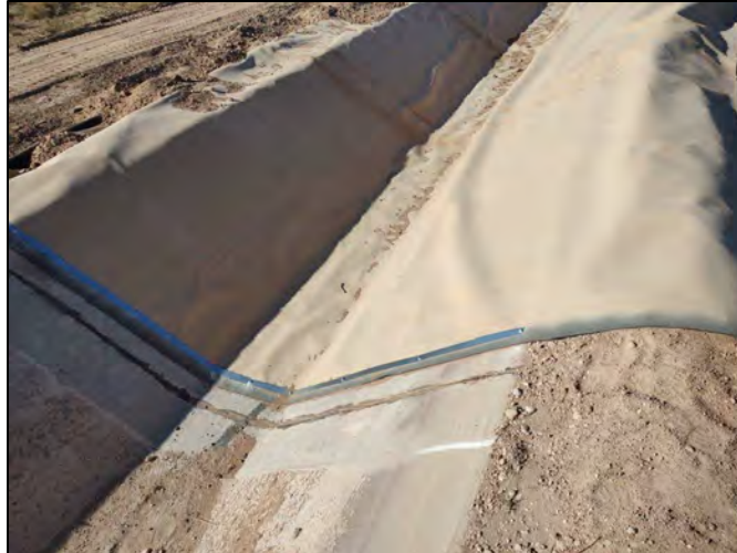
Figure 4. Photo of liner attached to existing concrete lining north of Lateral 26.5.
