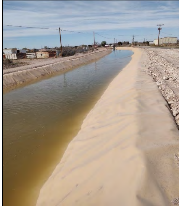
Figure 3. Photo of AssetGuard's Groundguard liner installed in CID's Main Canal.
