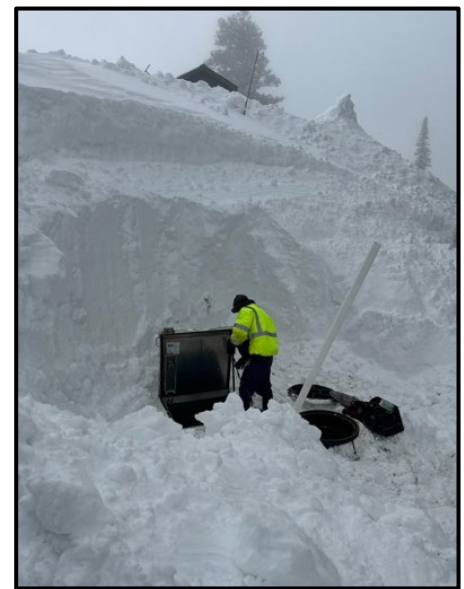
Figure 4: Digging to Find a Leak
