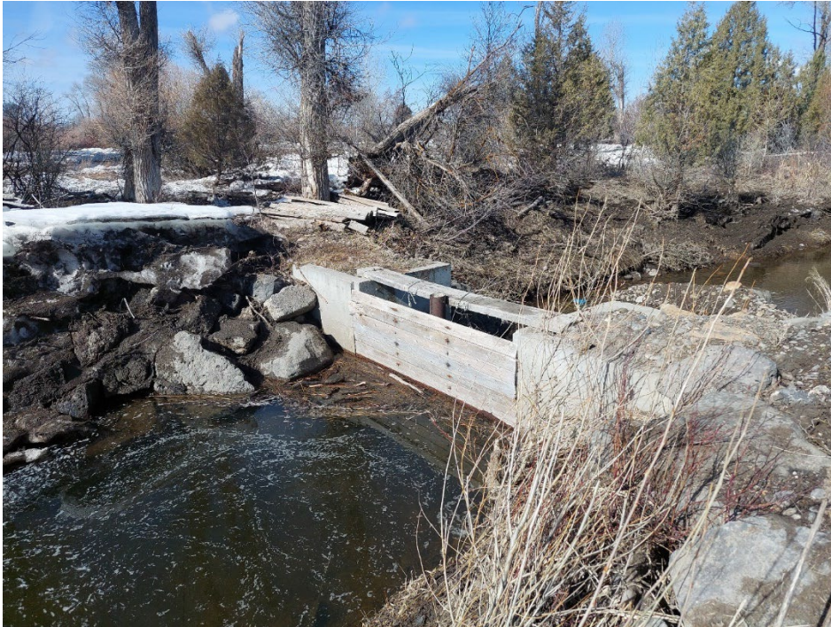
Figure 6-Existing SCC Headgate to be Replaced and Automated
