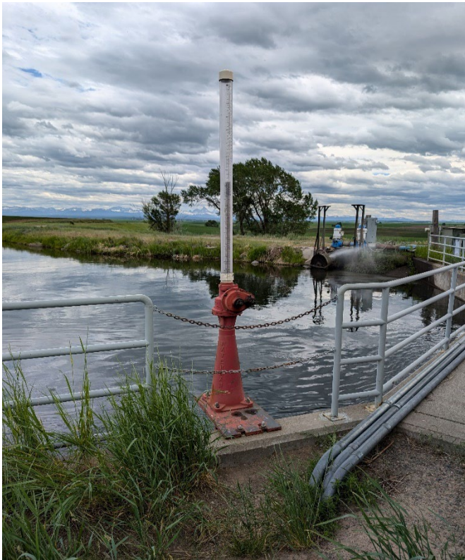
Figure 3-Marysville Canal Penstock-Gate to be Automated
