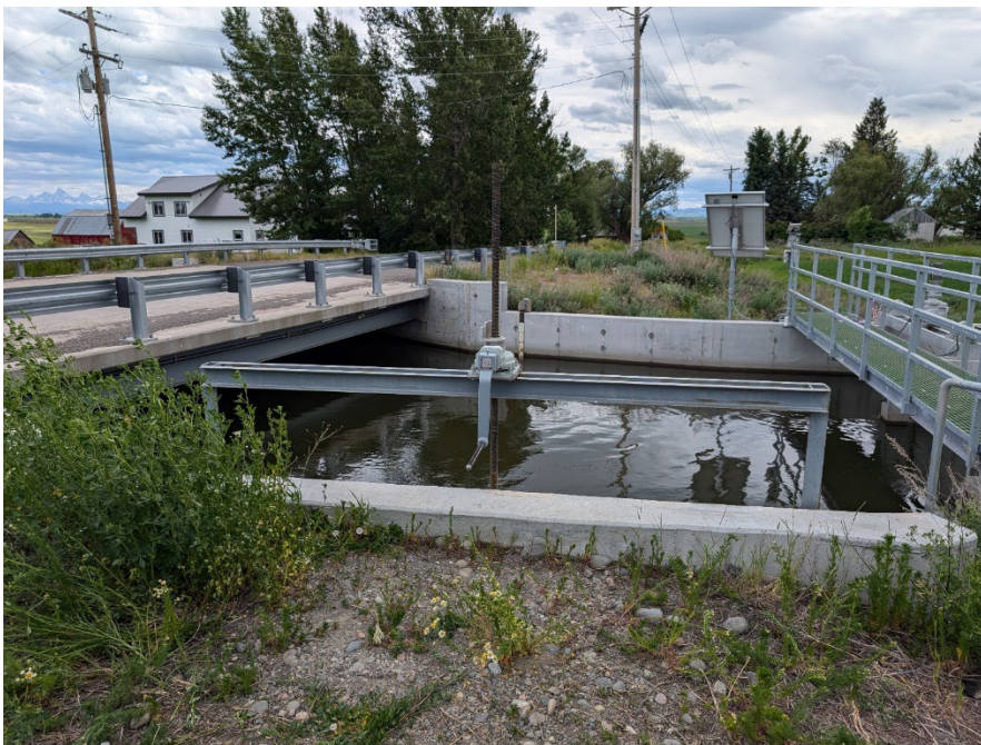
Figure 2-Kirkham Structure, Gate to be Retrofitted with Automation
