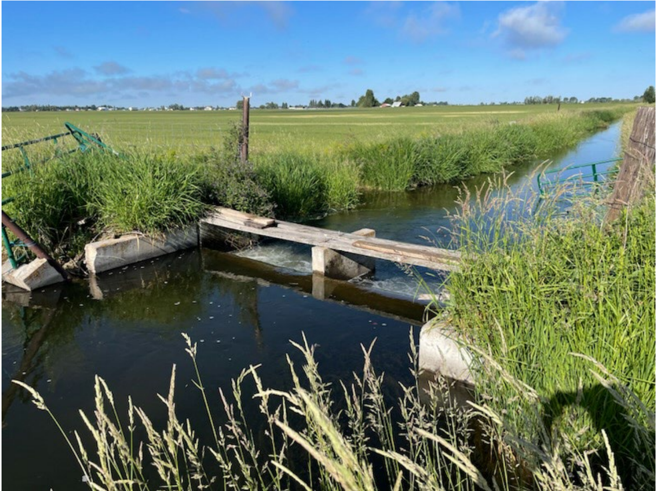
Figure 5-Structure 1, SICC-Fall River Canal Check Structure to be Retrofitted with Automation
