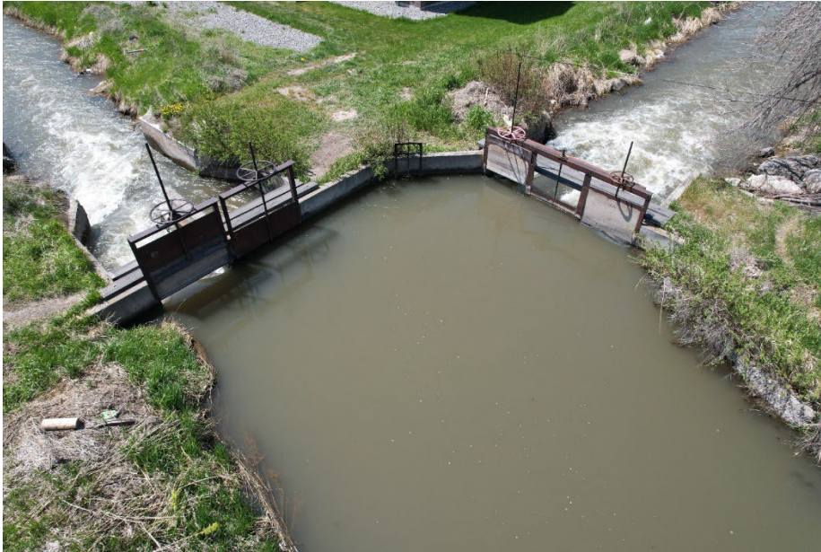
Figure 1-RICC Gates to be Retrofitted with Automation
