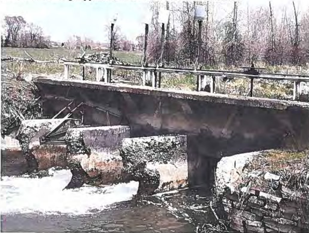
Picture 1: Existing support walls for main diversion structure
