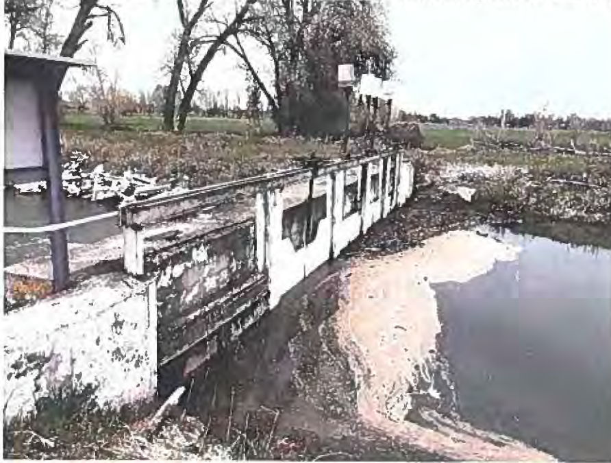
Picture 4: Gates – two in the middle have automation, two on the end have hand cranks
